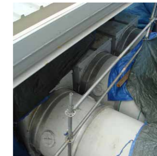
3 Welding connection in circuit breaker.
