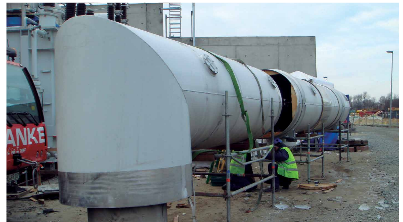
1 Welding connection between dilatation pieces
