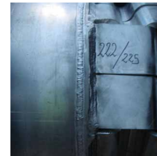
1 Welding connection between dilatation pieces
